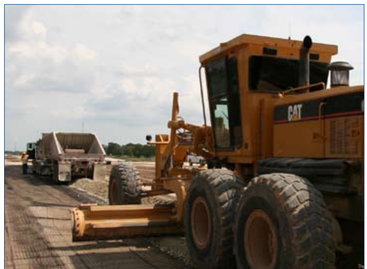
Photo 2: Belly dump spread over geogrids
