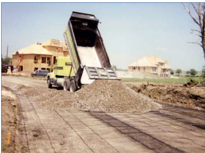
Photo 1: Back dump spread over geogrids
